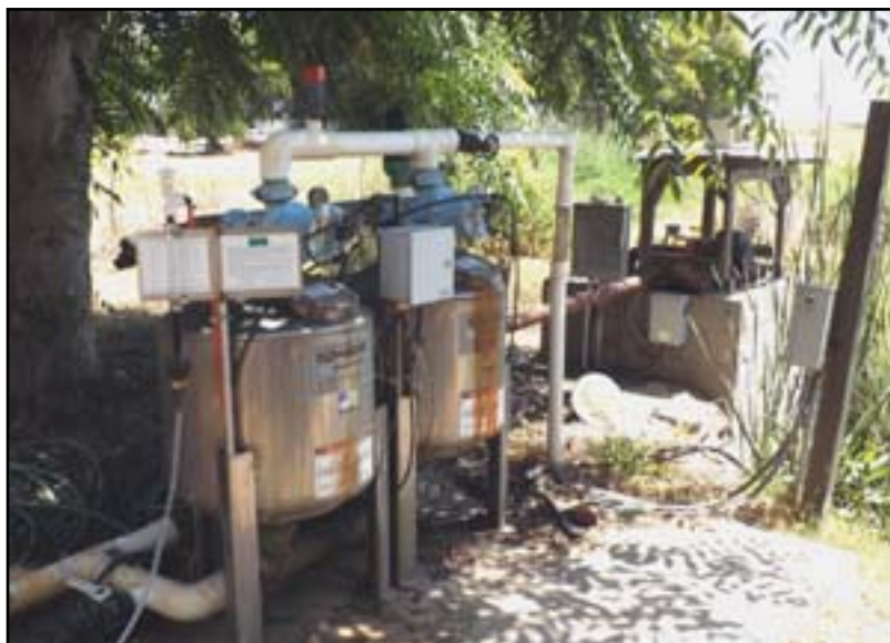
Fertigation system at the orchard of Harvey Correia in Isleton, CA.
